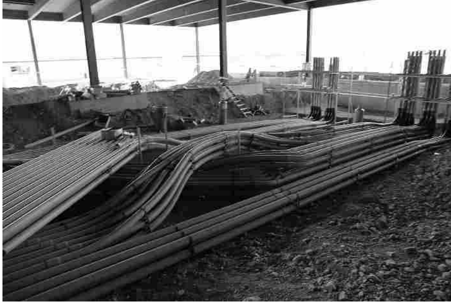
Figure 3.1.2: Underground PVC Conduit in Data Center Construction
